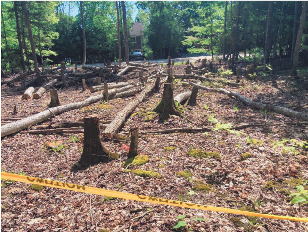
Photo No. 4: Tree clearing area looking east out to County Rd, Note flagging tape perimeter, May 2024
