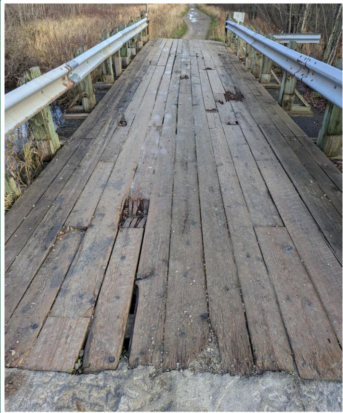
View of Structure Facing North
