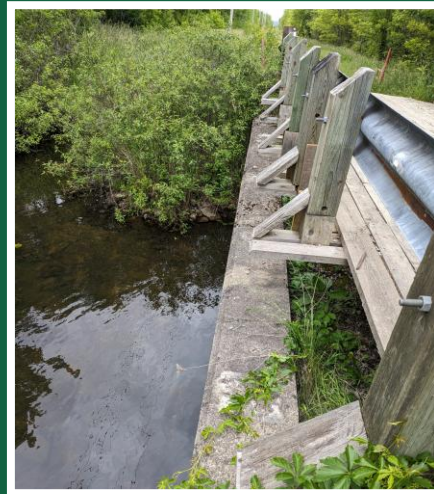
View of Barrier System
