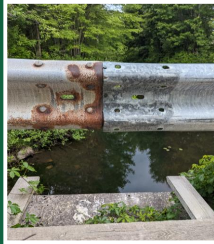
View of Barrier Lap Splice
