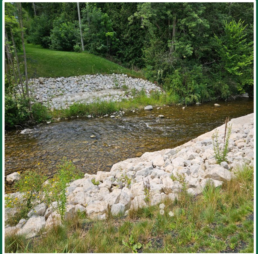
Photo example from Orchardville Bridge
