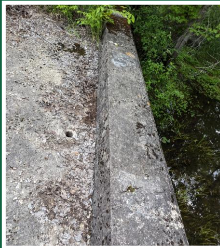
View of Concrete Curb and Deck Top
