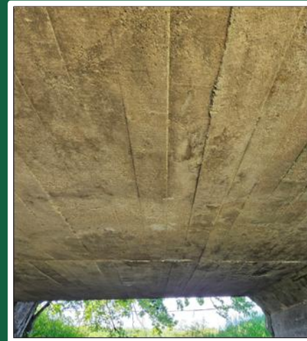
View of Interior Soffit
