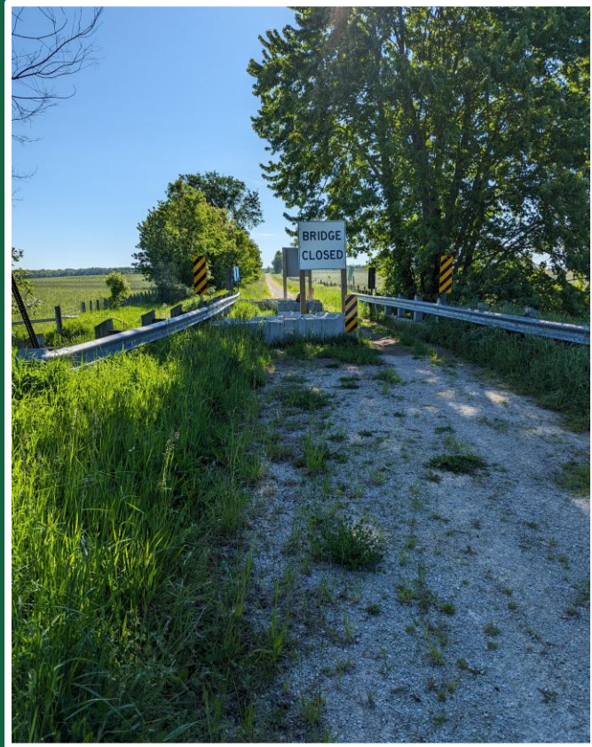
View of Structure Facing East
