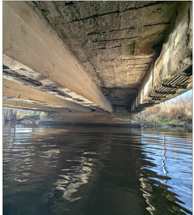
Photo 6 - View of Concrete Structure Interior Soffit.
