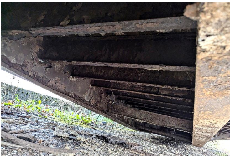
Figure 5.2: Typical Floor Beams
