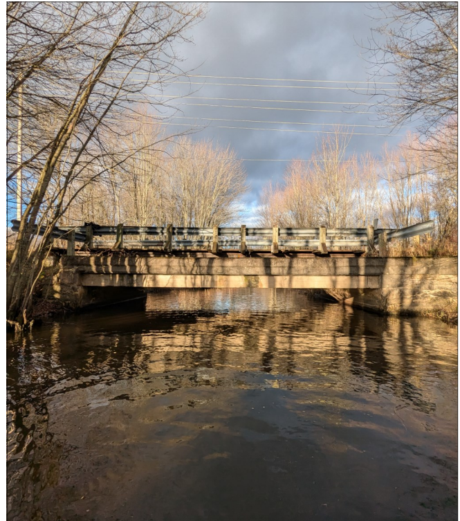
Photo 2 - View of Structure Facing West.
