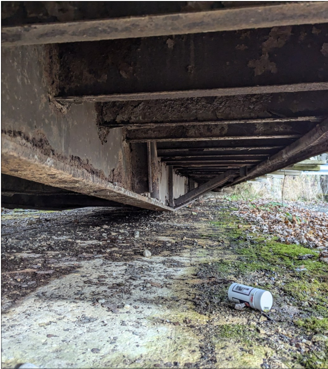
Photo 9 - View of Cantilevered Floor Beams.
