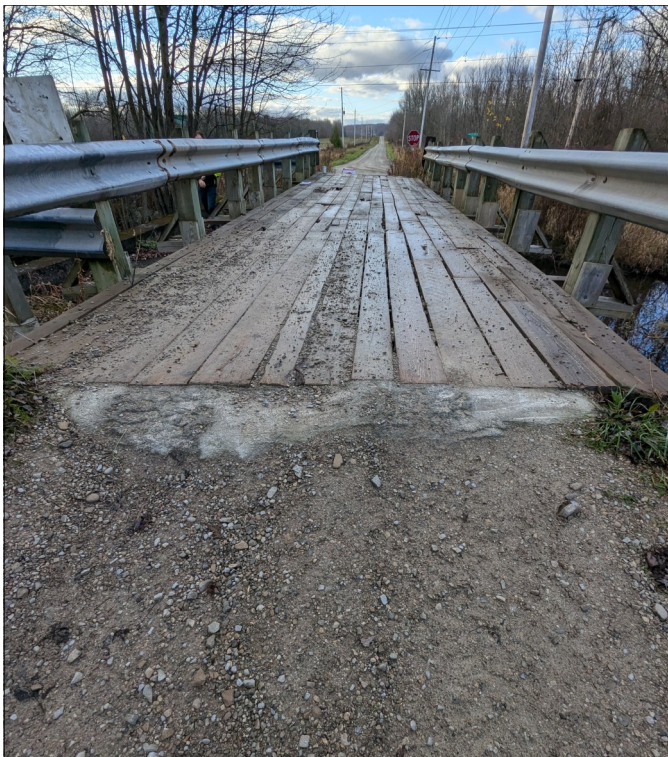
Photo 3 - View of Structure Facing South.
