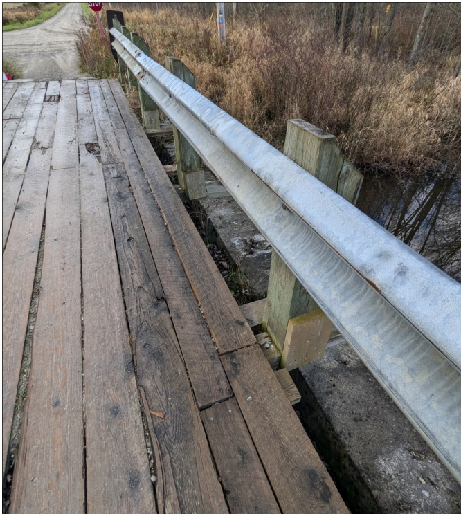
Photo 7 - View of Steel Beam Barrier System.
