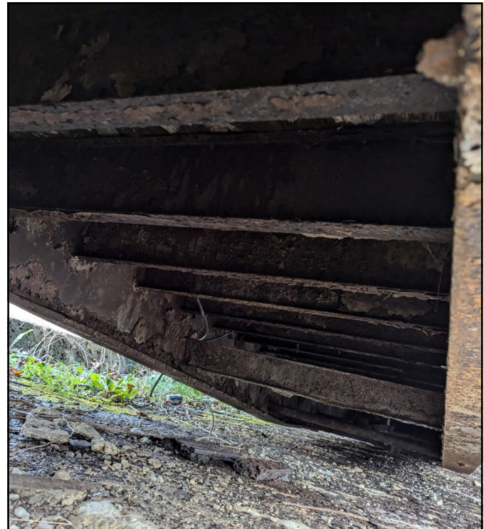
Photo 12 - View of Interior Floor Beams.
