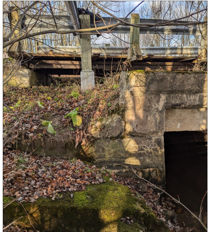
Photo 14 - View of Southeast Wingwall of Original Structure.
