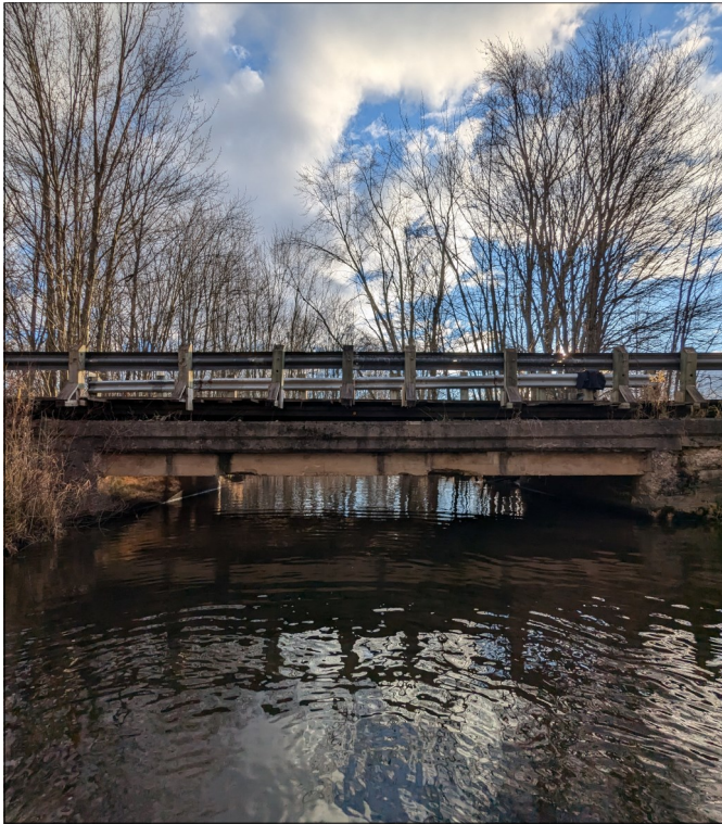
Photo 1 - View of Structure Facing East.
