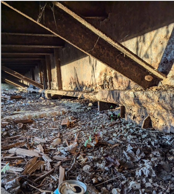
Photo 11 - View of Steel Girder and Diagonal Strutting.
