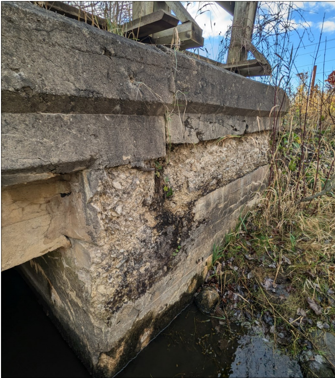
Photo 13 - View of Southwest Wingwall of Original Structure.
