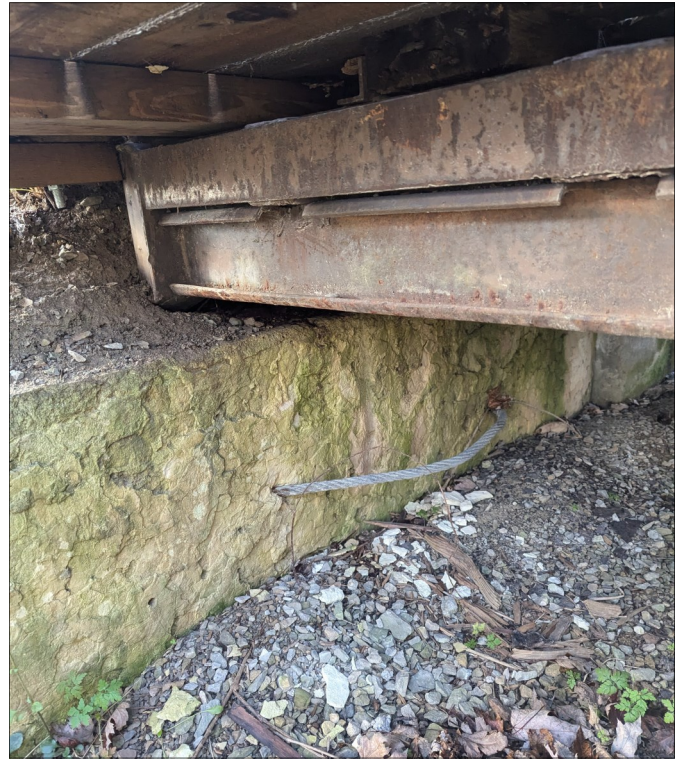
Photo 10 - View of South Concrete Abutment.
