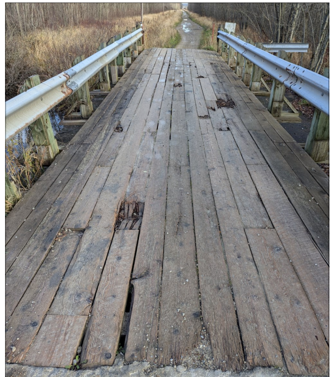
Photo 4 - View of Structure Facing North.
