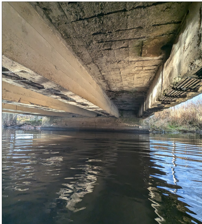
Photo 15 - View of Interior Soffit of Original Structure.
