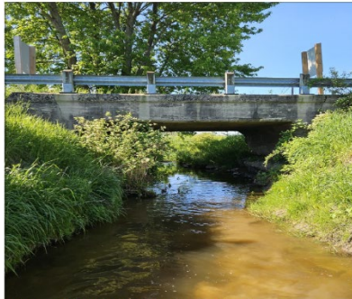
Photo 1 - View of Structure Facing South
