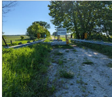
Photo 2 - View of Structure Facing East.
