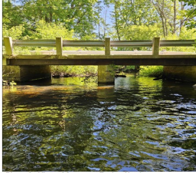
Photo 2 - View of Structure Facing North.
