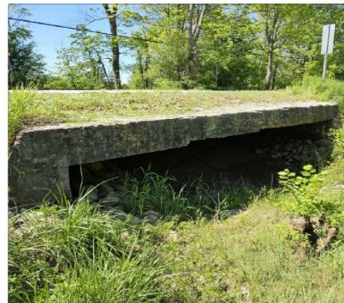
Photo 2 - View of Structure Facing South.
