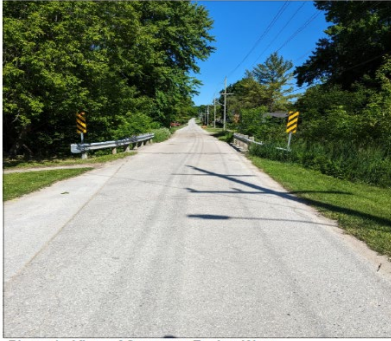
Photo 1 - View of Structure Facing West.
