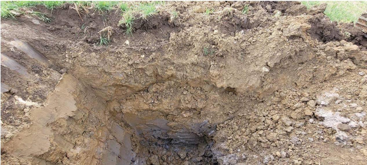
Picture 21: TH-07 – Side view showing soil profile.
