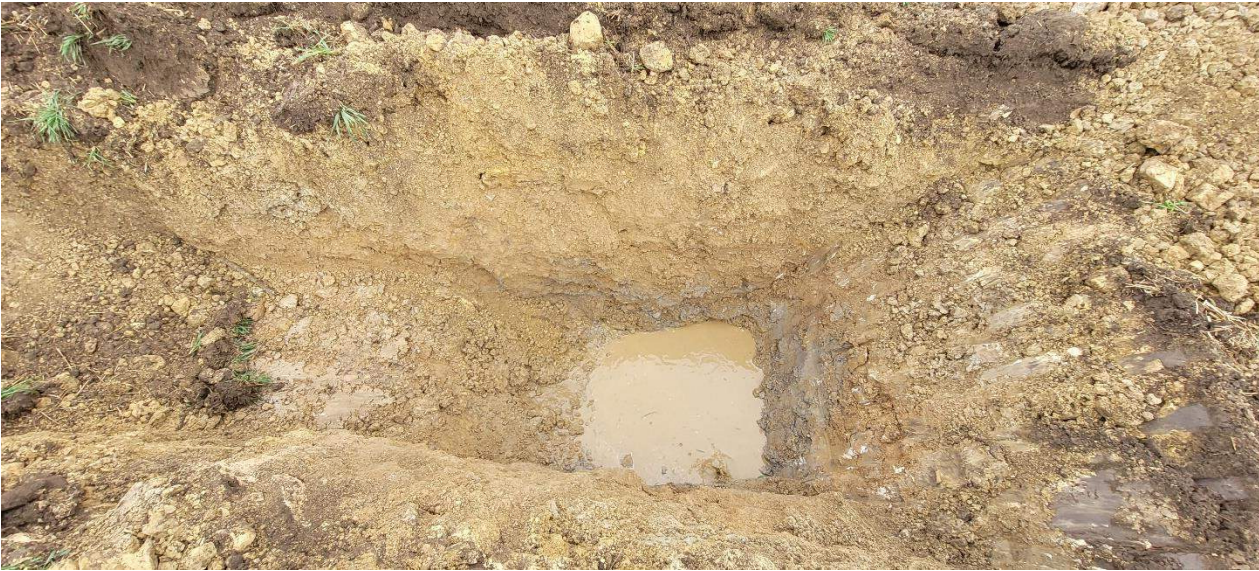
Picture 10: TH-04 – Overhead view.
