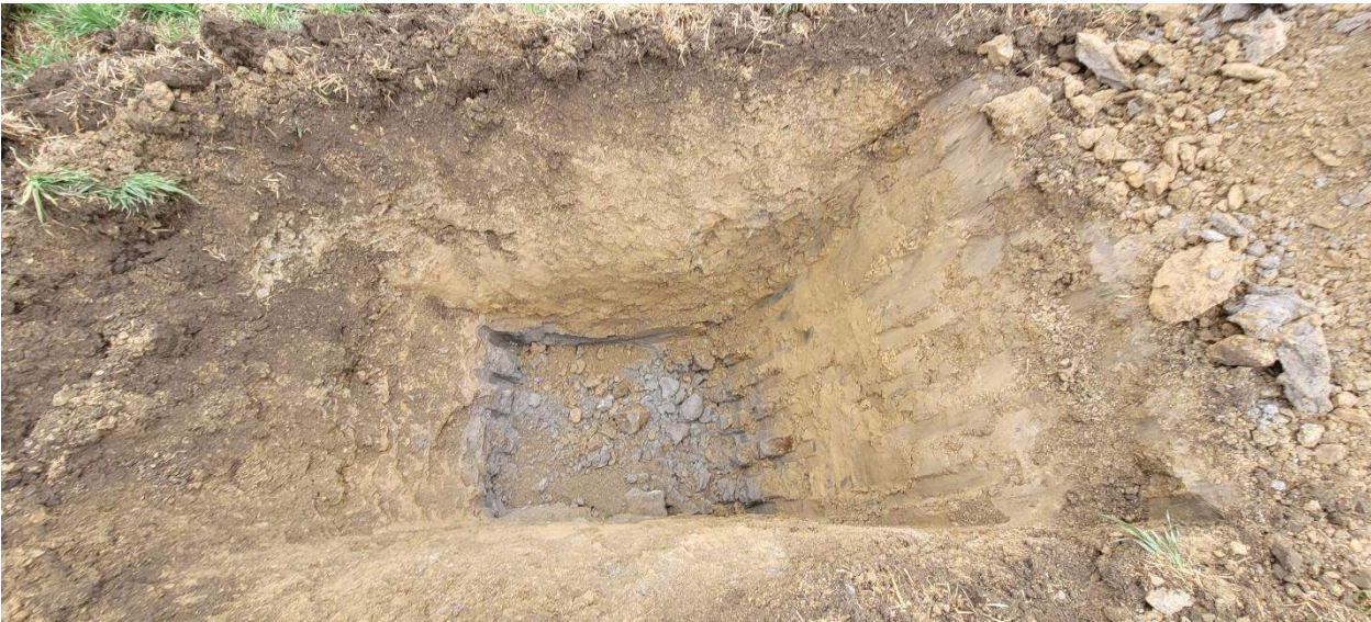
Picture 7: TH-03 – Overhead view.
