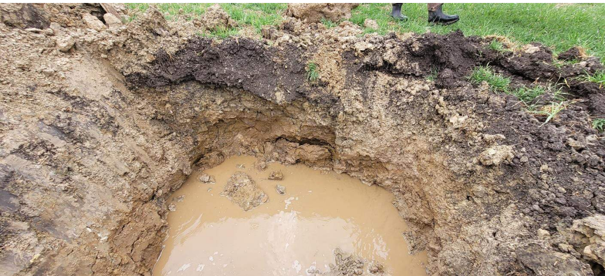
Picture 6: TH-02 –Side view showing soil profile.
