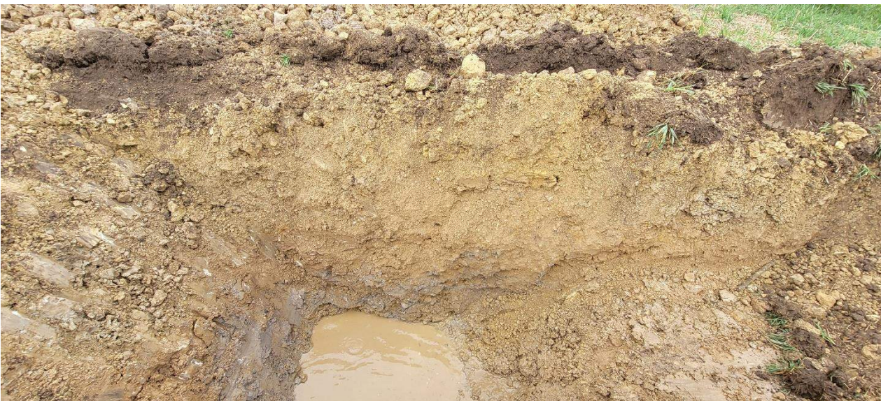
Picture 12: TH-04 – Side view showing soil profile.
