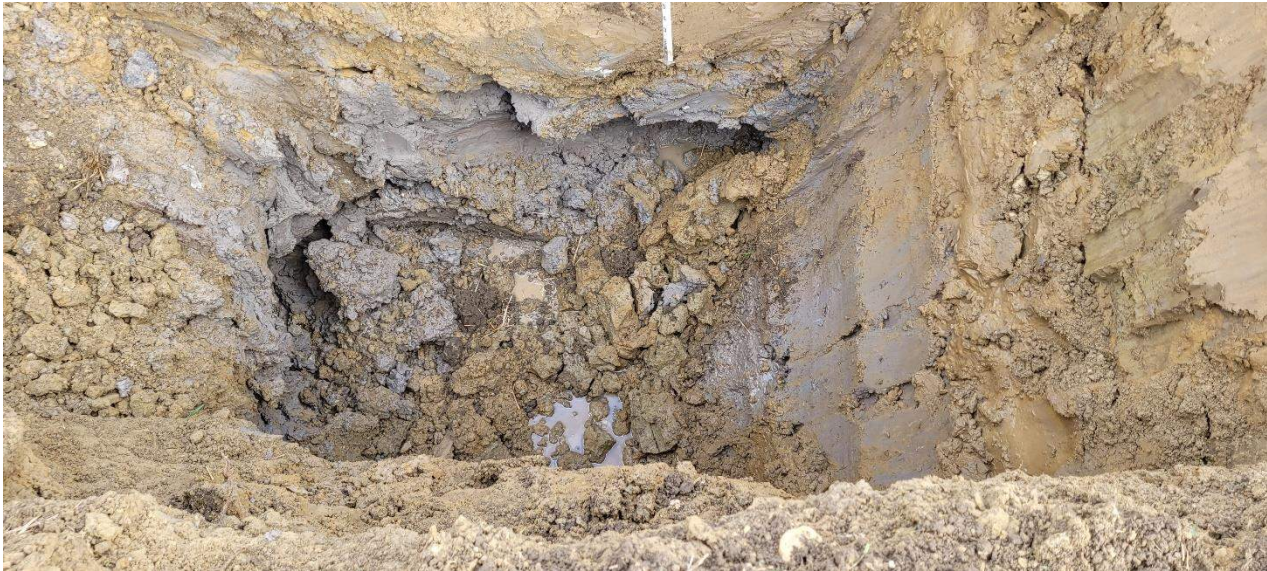
Picture 20: TH-07 - Close up view of testhole bottom.
