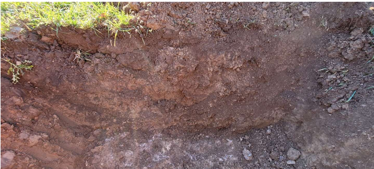
Picture 12: TH-04 – Side view showing soil profile.
