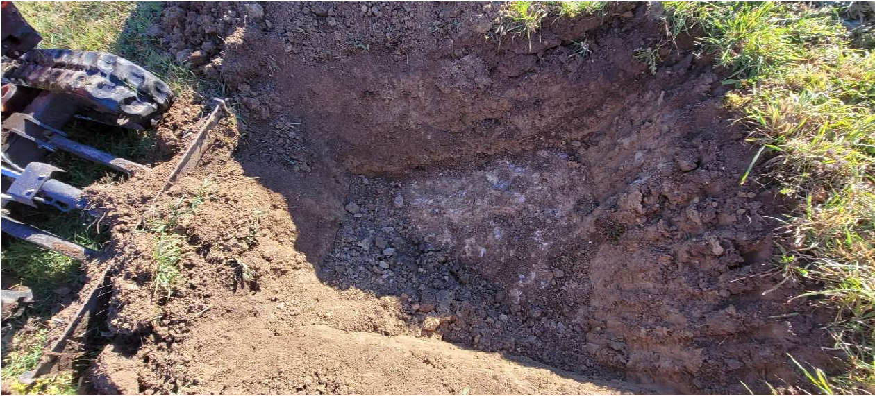
Picture 10: TH-04 – Overhead view.
