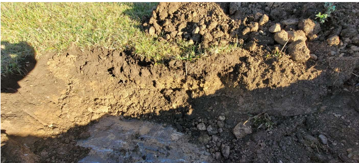
Picture 3: TH-01 – Side view showing soil profile.
