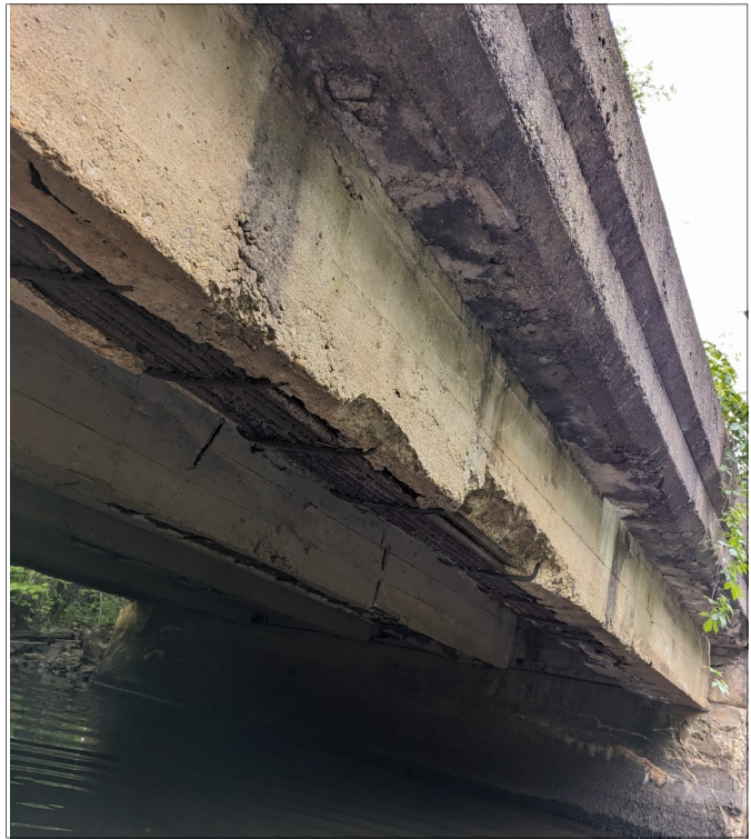
Photo 10 - View of Underside of Lower Structure.
