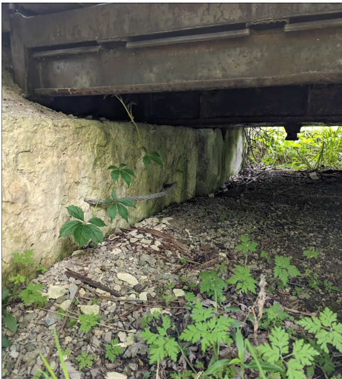
Photo 7 - View Upper Structure Abutment Wall.
