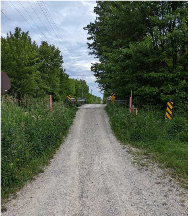
Photo 1 - View of Structure Facing North.
