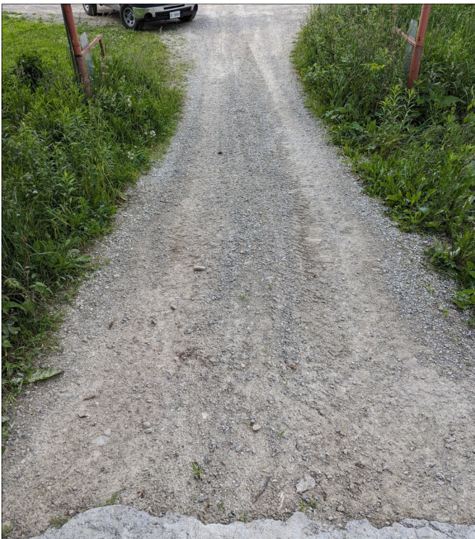
Photo 15 - View of Steep Gravel Approach.
