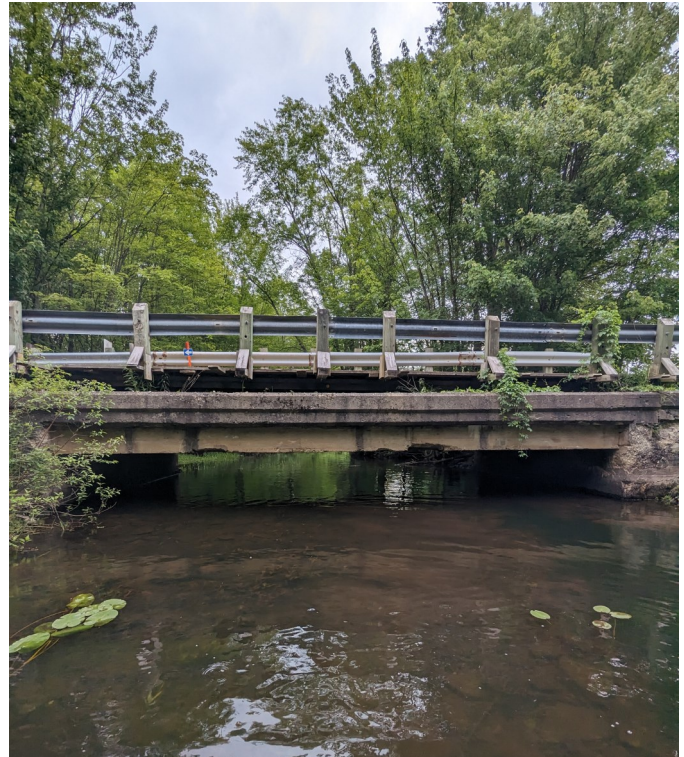
Photo 2 - View of Structure Facing East.
