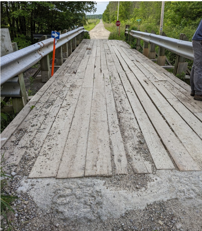
Photo 3 - View of Deck Top (Upper Structure) Facing South.
