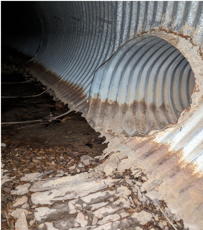
Photo 9 - View of Storm Pipe Connection at North Barrel.
