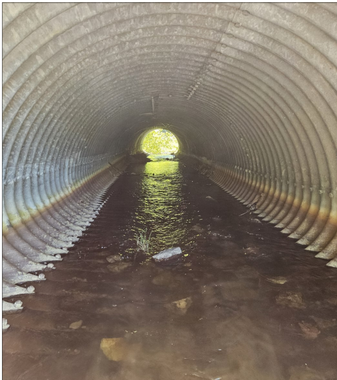
Photo 3 - View of Barrel Facing East.
