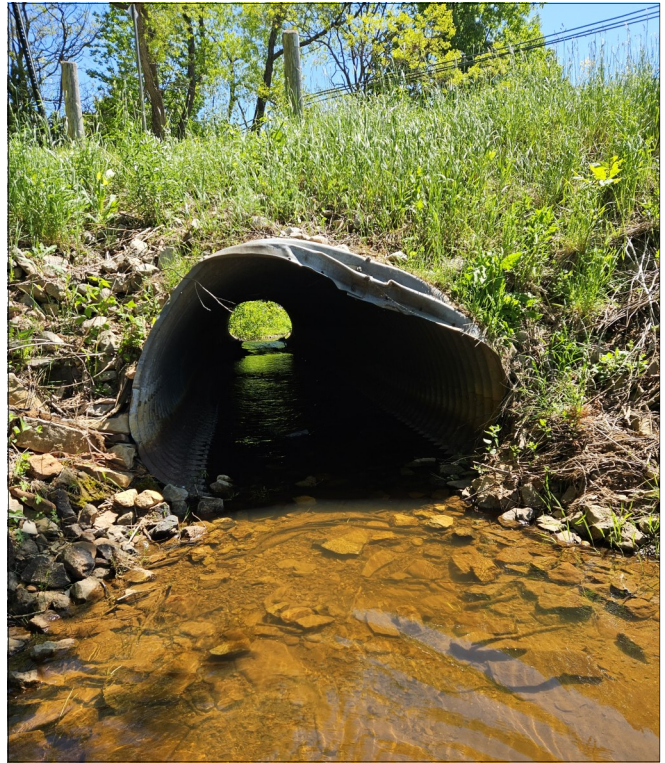
Photo 2 - View of West Culvert End.
