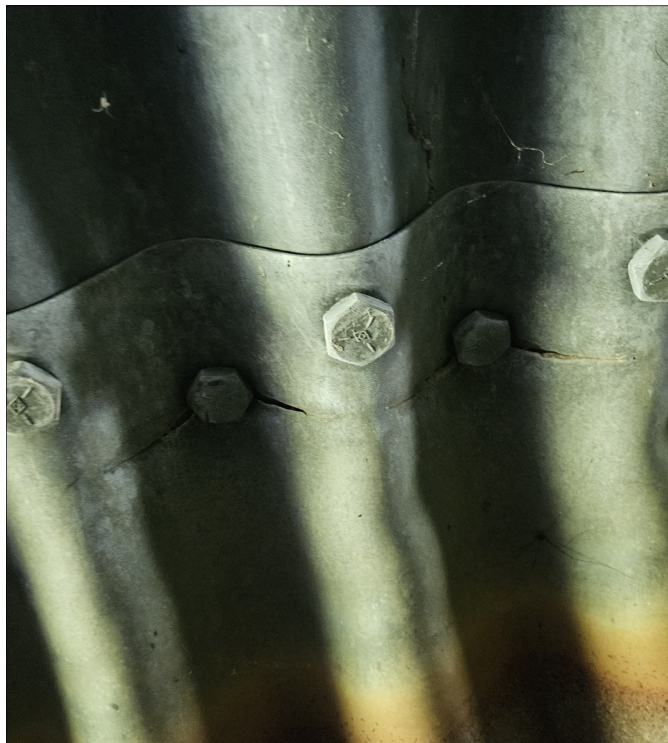
Photo 7 - View of Bolt Hole Cracking on South Wall of Barrel.
