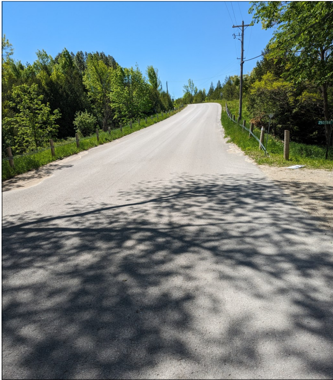
Photo 1 - View of Structure Facing South.
